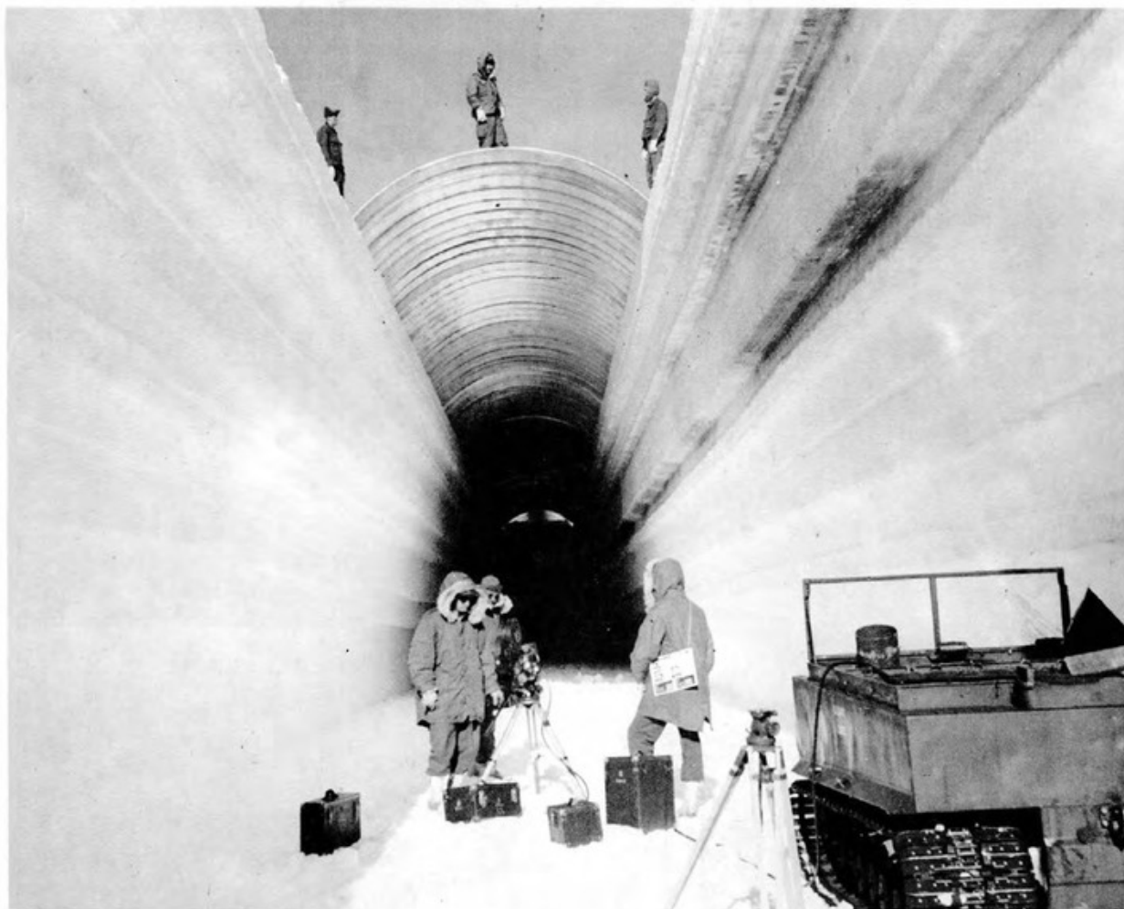
Figure 14. Metal arch forms being emplaced over undercut trench.
