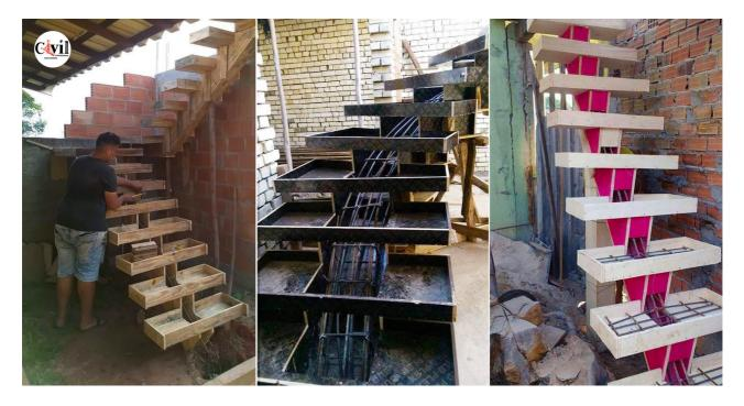
A stair stinger is a structural member that is installed on either side or at the center of a flight of stairs with threads and risers fixed. The primary function of the stringer is to provide a framework or support to the tread & risers and to hide the edge of the stairs exposing the tread profile.
